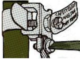
■ The earth tags (above right) should be connected to all pipes and can be bought from most diy stores and electrical merchants. They are proprietary connections reading **ELECTRICAL CONNECTION DO NOT REMOVE**.
